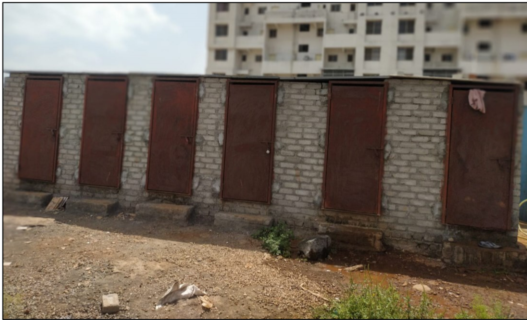
Photographs of Toilets for Labor at Site
