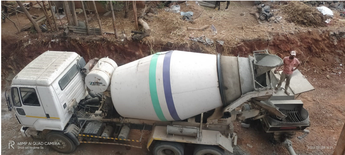
Photographs of Use of RMC Machine at Project Site
