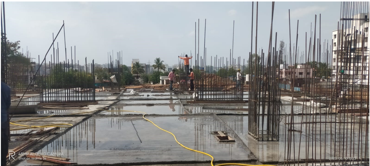
Photographs showing Curing practice at site
