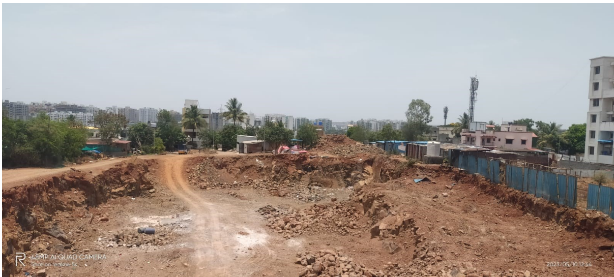
Excavation on site
